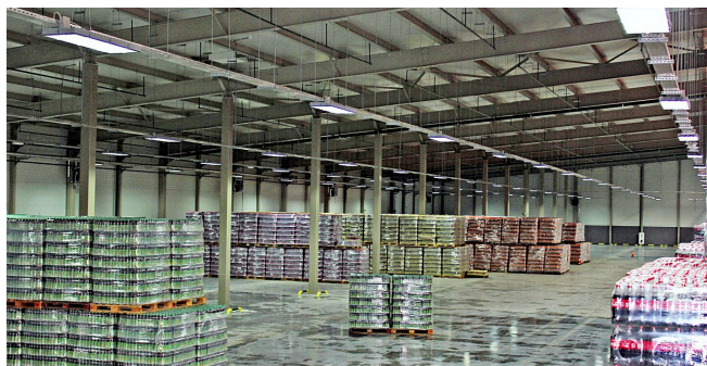
DISTRIBUTION HALL · BISHKEK
