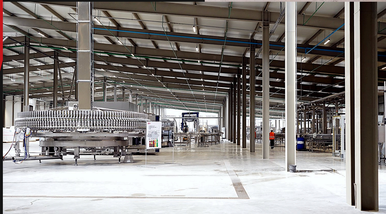
PRODUCTION HALL — COCA-COLA PLANT, SHYMKENT
